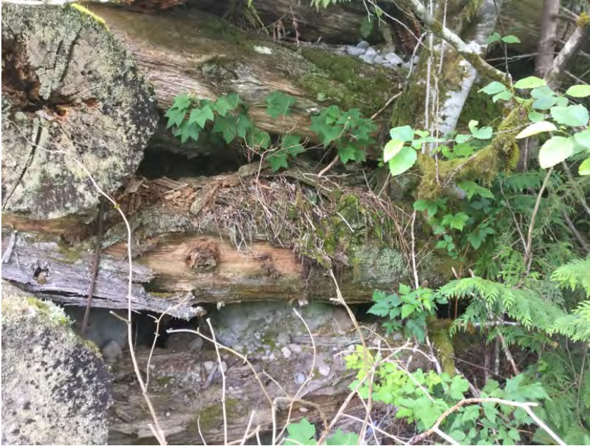
Downstream left bank wingwall
