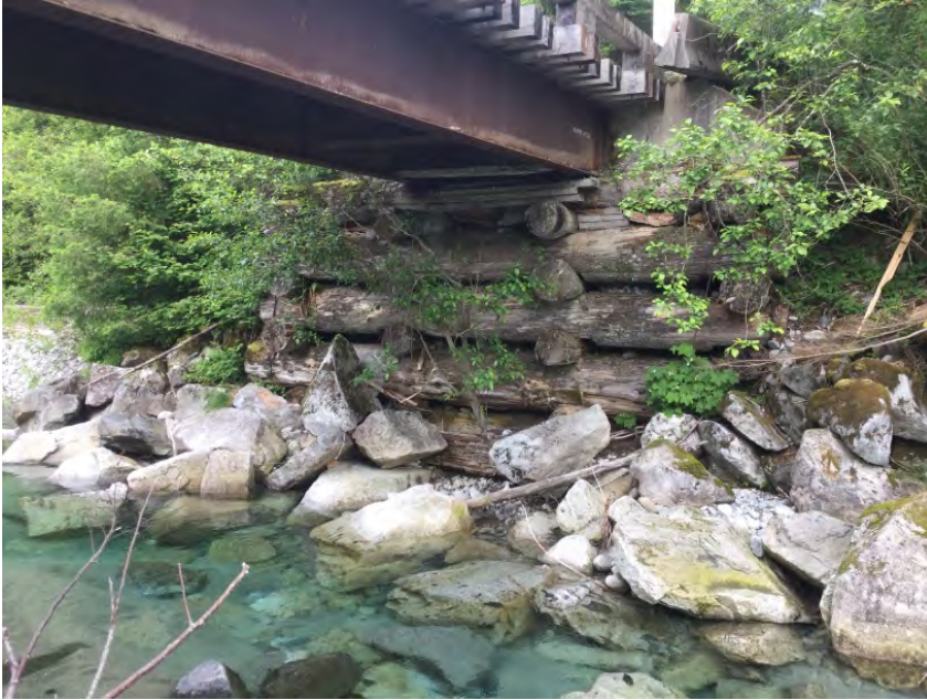
Right Bank Abutment when facing downstream
