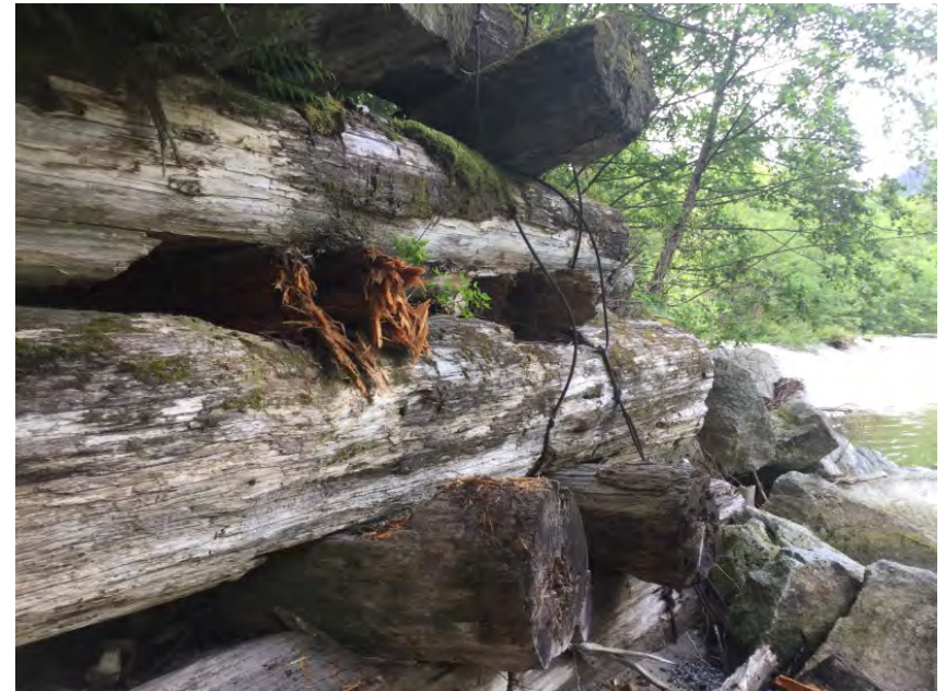
Tieback condition on left abutment
