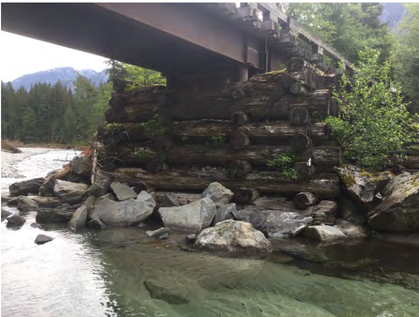
Right side of pier
