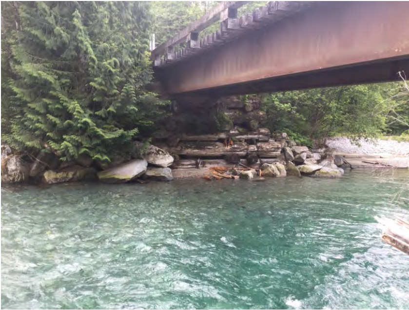
Left Bank Abutment when facing downstream
