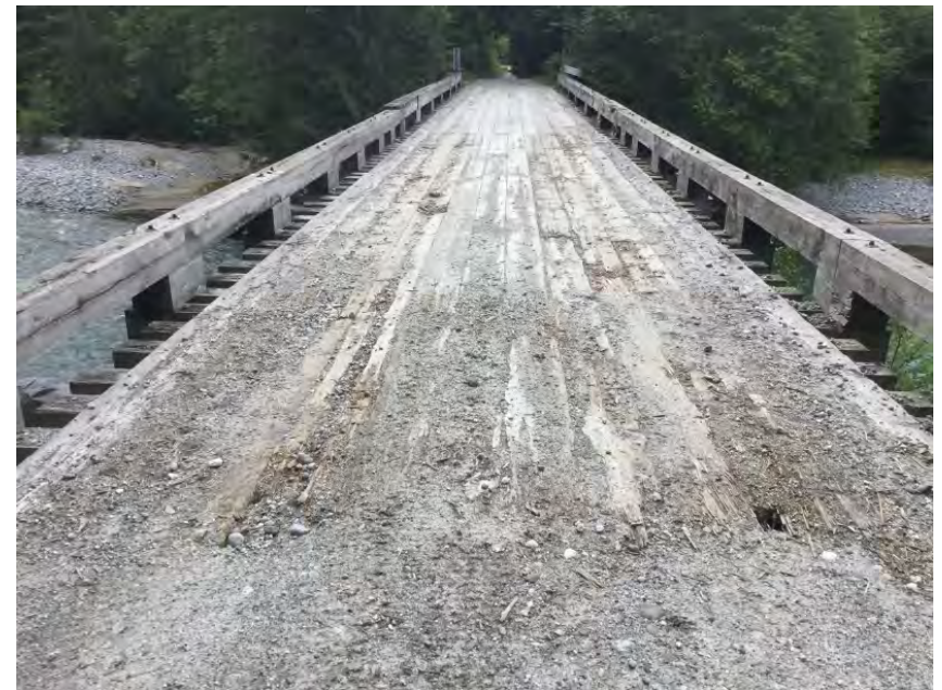
Right span deck condition
