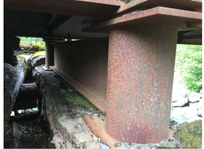
Right side of pier
