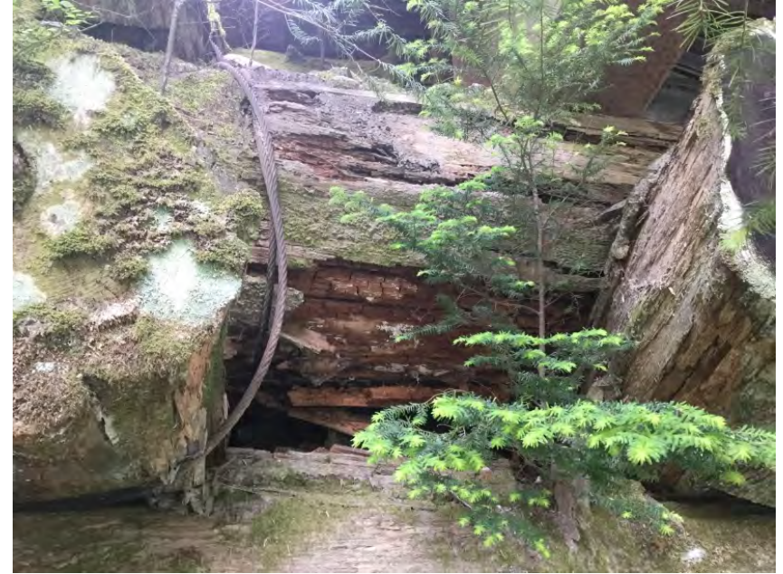
Top crib log on left abutment
